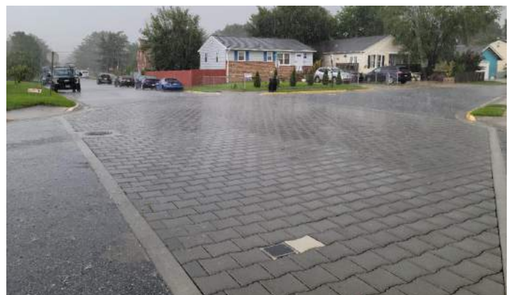
Completed site during rain 2022
