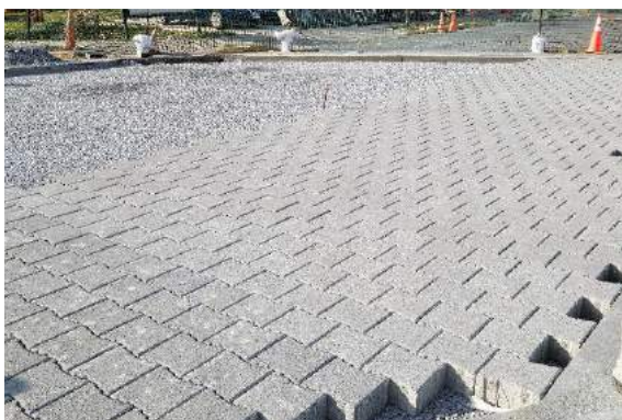
Placement of PaveDrain surface
